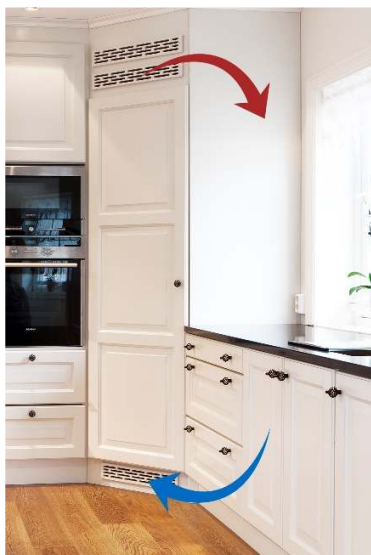
Kitchens built to ceiling height must have air vents installed in both the header and footer boards
