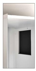
When the base and panels are in perfect position, lift the roof section on top of the fridge walls, line up carefully, and use the allan key to lock the section in place.
