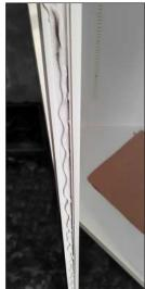
Apply silicone across the front of the roof section, and across the front of the base.
