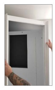
Rotate the frame to make sure the hinge is on the correct side.
