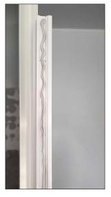
On the inside of the frame, use silicone sealant down both sides where the fridge wall and door frame meet.
