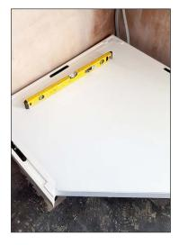
Position the fridge base in to the corner, leaving a space of around 45mm along the right hand wall, but close up to the left hand wall.
