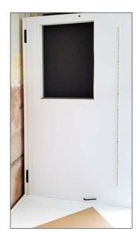
When the fridge base is perfectly level, and the gap along the right side of the base is 45mm from the wall, the first panel can be installed.
